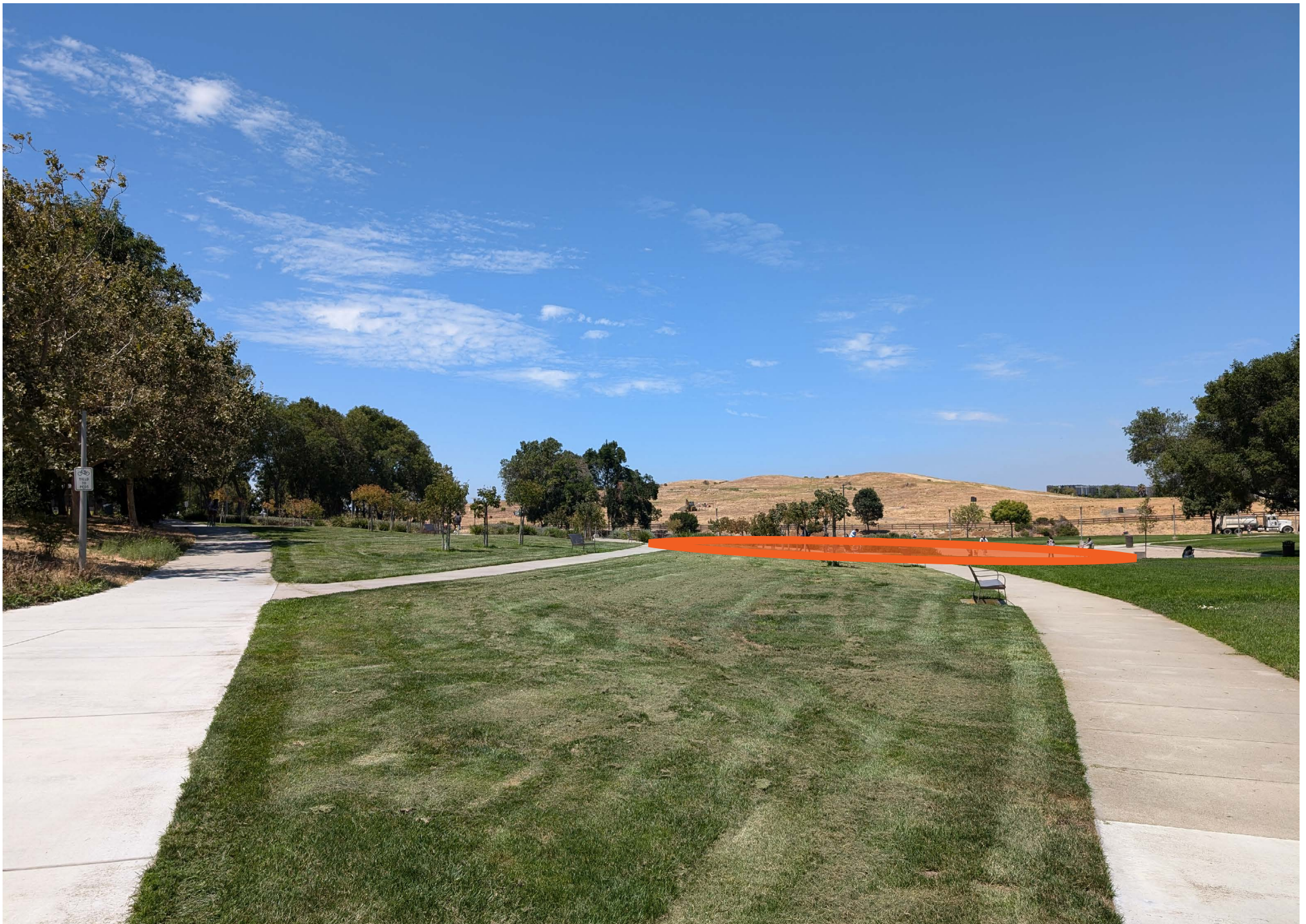
Camera Location "D", View Towards Reservoir Underground Reservoir Location
