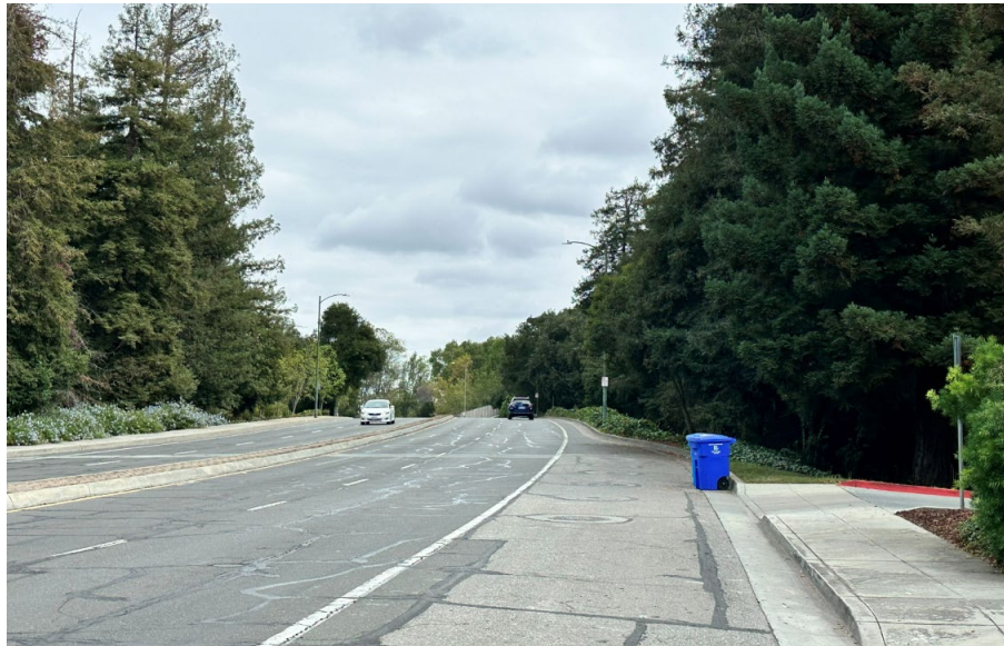
Figure 5: Sidewalk terminates at 555 W Middlefield Road (eastbound)
