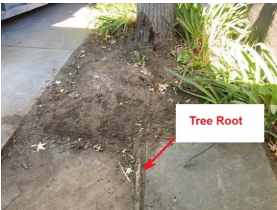
Photo No. 4 (Tree No. 2)—Photos of root damage to pathway adjacent to Tree No. 2
