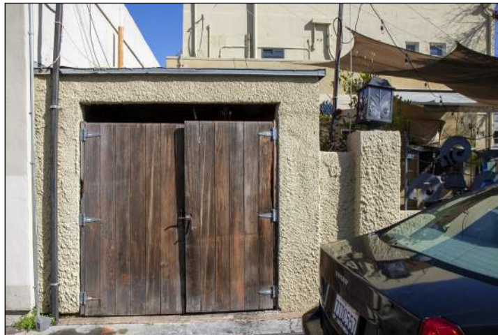
Shed at northwest corner added ca. 1983.
