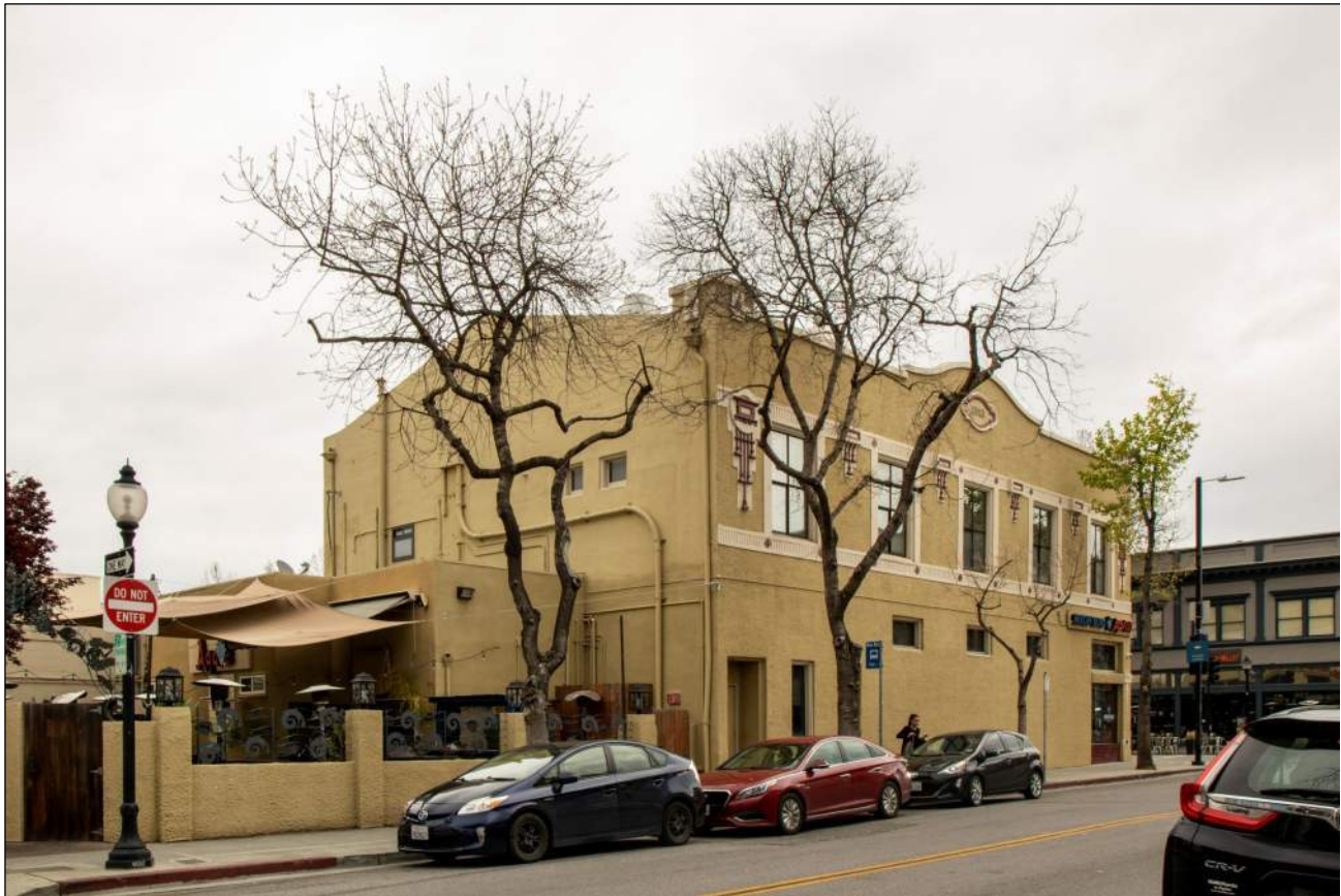
Southwest corner of Jurian Building showing the southern and western elevations, wall built ca. 2000, and part of the lower-story extension that was added between 1921-1943. Viewed with camera facing east.
