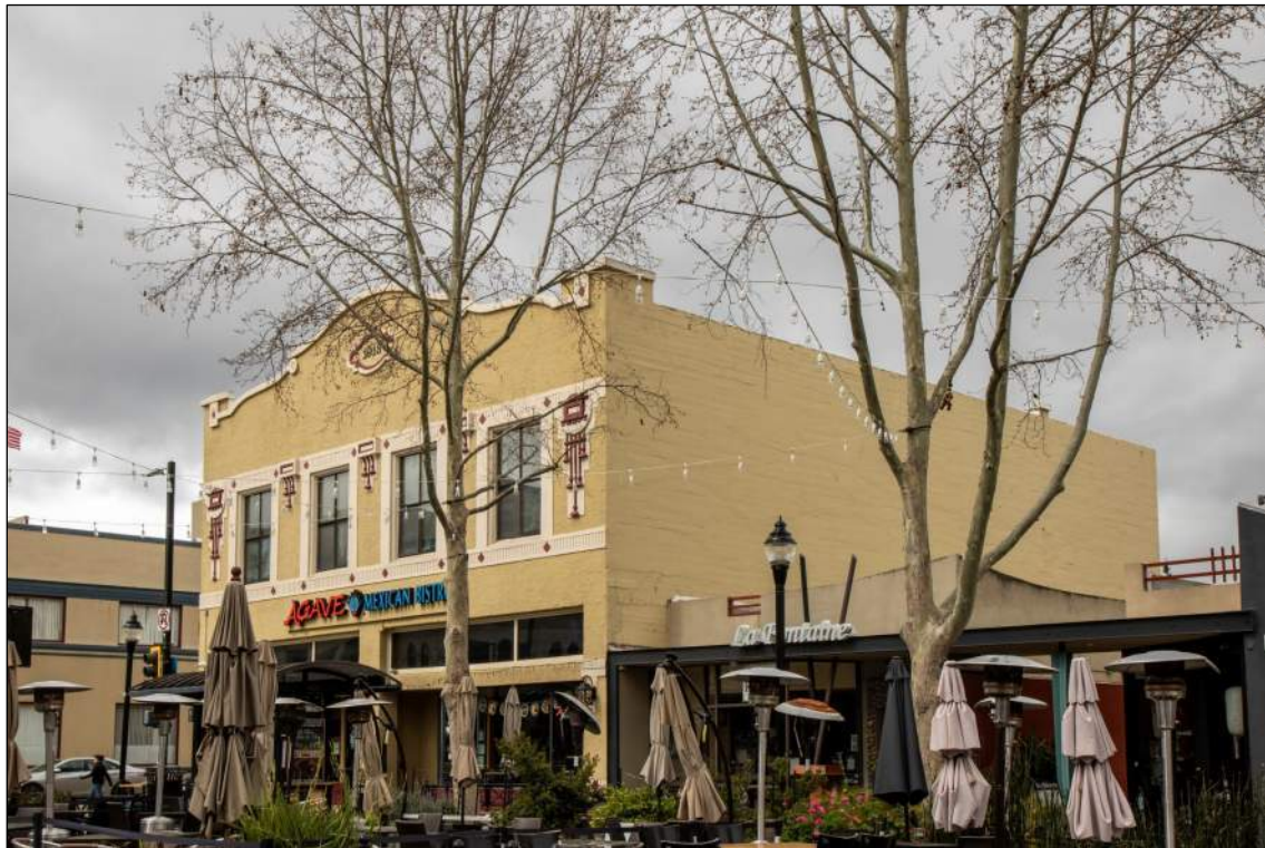
Northern facade of Jurian Building.
