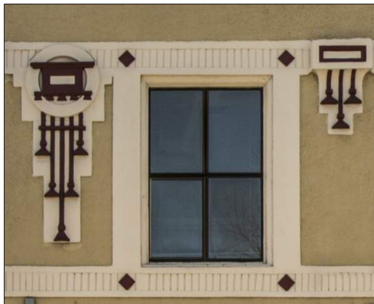
Closeup of window and decorative moldings.
