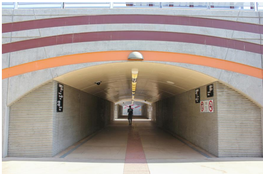
Figure 7: Santa Clara Caltrain Station Undercrossing
