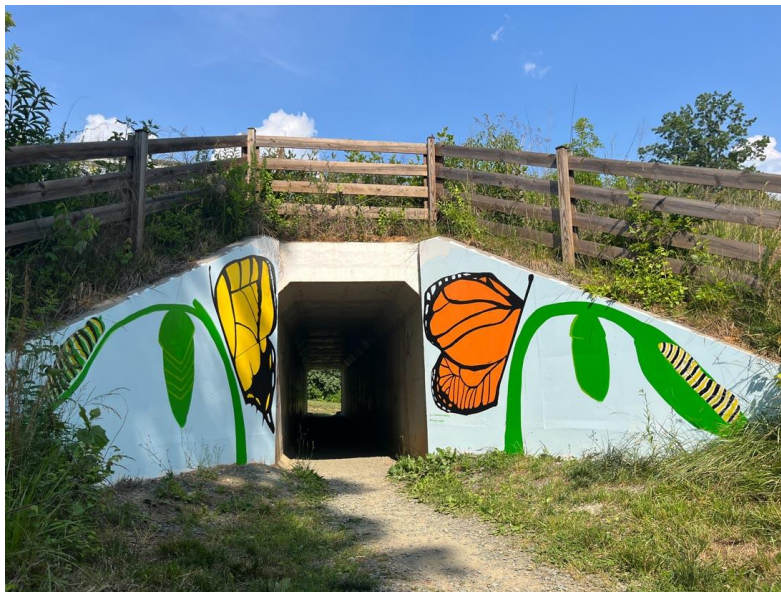
Figure 6: Painted Retaining Wall
