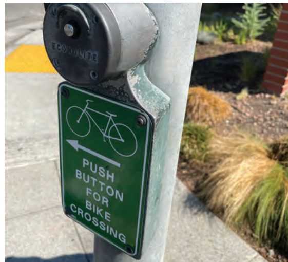
Bicycle push buttons allow bicyclists to request a green light
