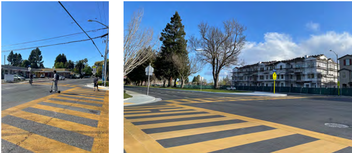
FIGURE 15 MARKED CROSSWALKS IN MOUNTAIN VIEW
