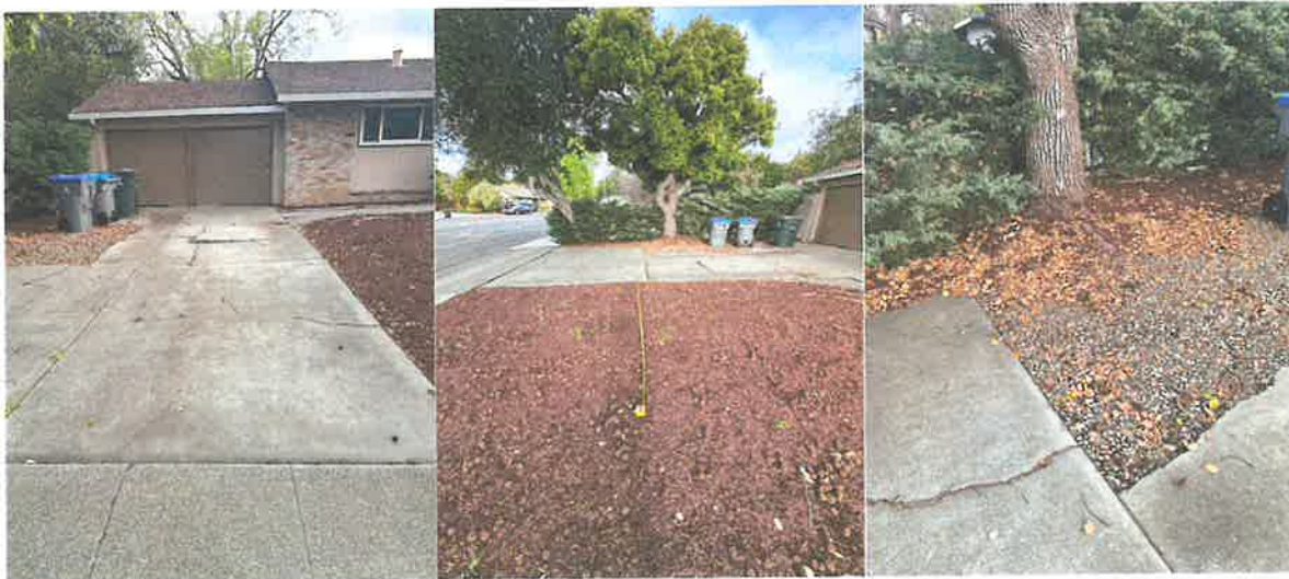
Figure 8,9,10: Existing driveway damage
