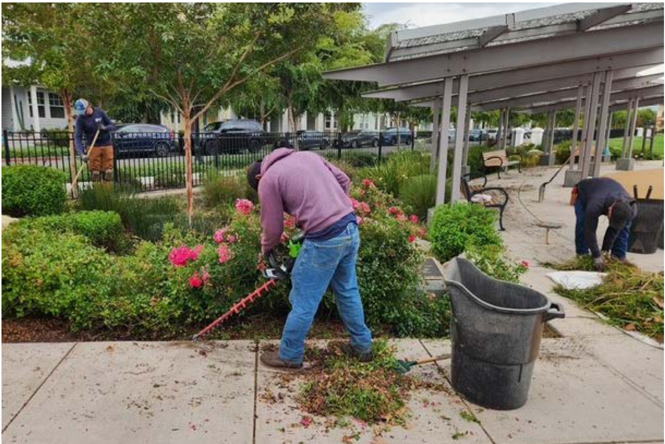
Routine maintenance of bioretention system at Pyramid Park. Photo courtesy of the City of Mountain View.
