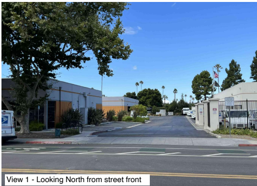
View 1 - Looking North from street front
