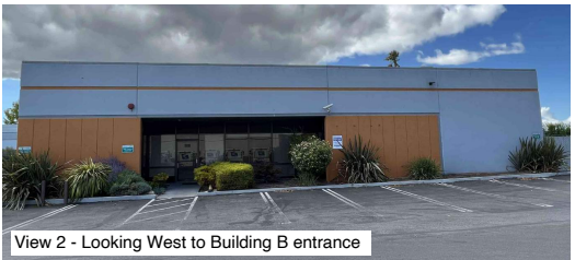
View 2 - Looking West to Building B entrance
