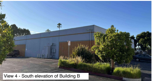
View 4 - South elevation of Building B
