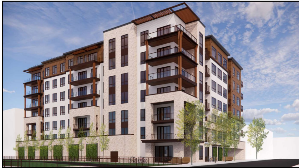
Figure 3: View of the Project from the East Along Fayette Drive
