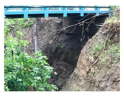
Figure 2: Sleeper Avenue Bridge Bank Erosion
