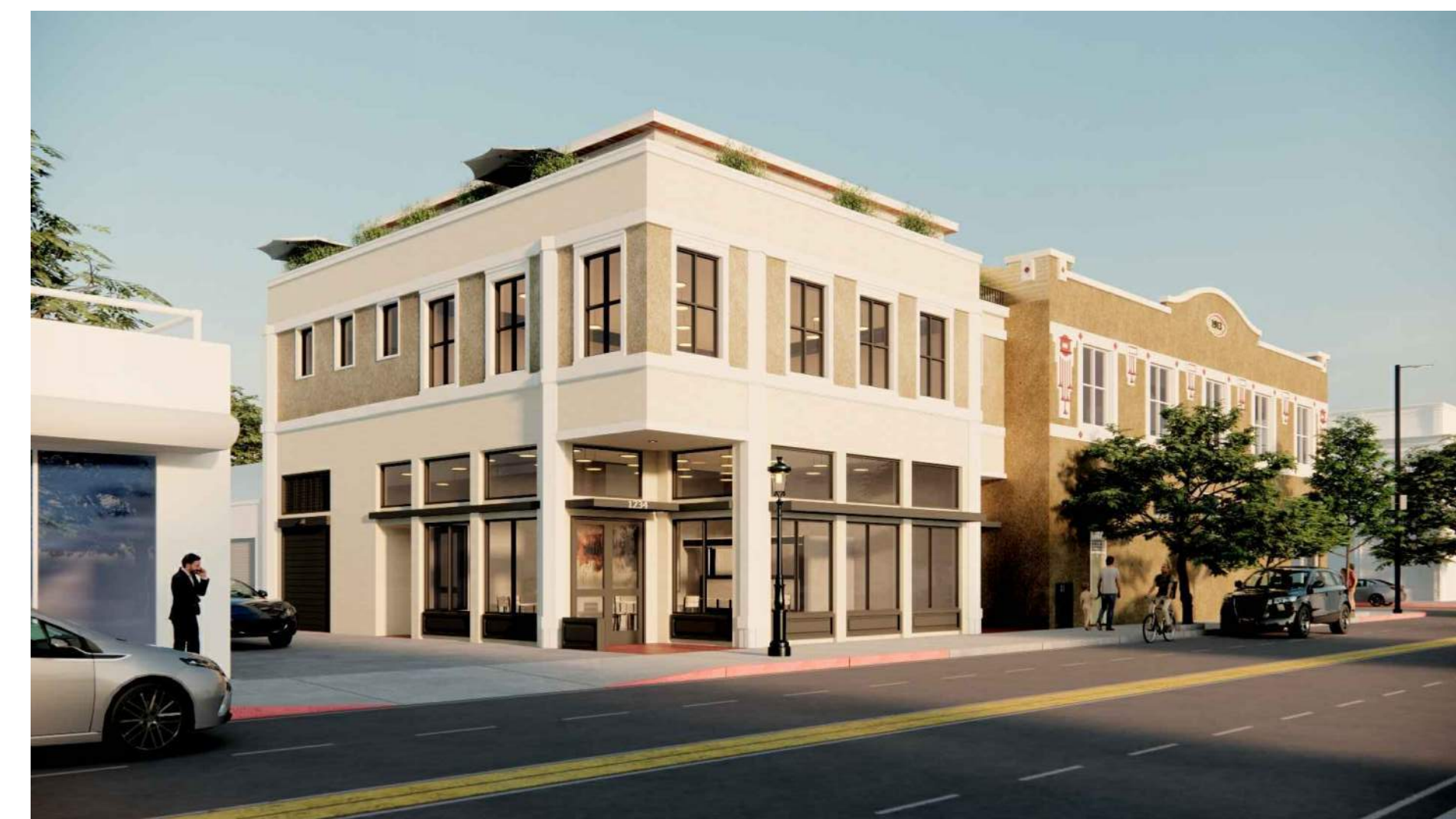
B VIEW FROM VILLA STREET LOOKING NORTHEAST
