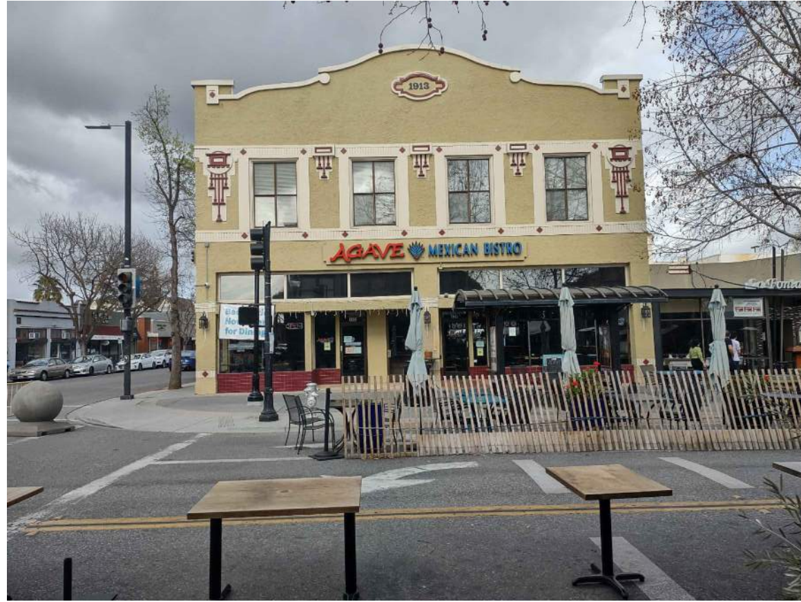
1 PHOTO FROM CASTRO ST., LOOKING WEST
