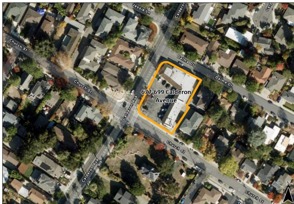
Figure 5: 677-699 Calderon Avenue Existing Conditions
