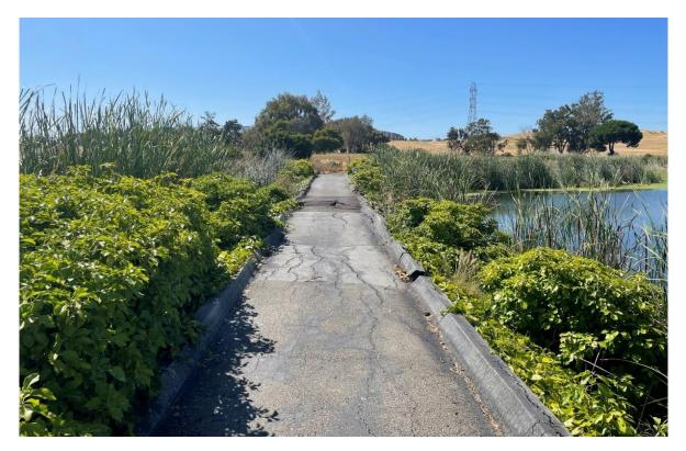
Photo 1. View of Existing City Bridge #25 looking southeast across the top of the existing deteriorated causeway.<sup>1</sup>
