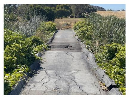
Photo 2. Closeup of existing deterioration Bridge #25.
