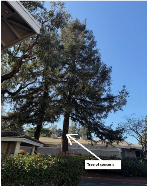
Photo #2 Driveway view of tree of concern
