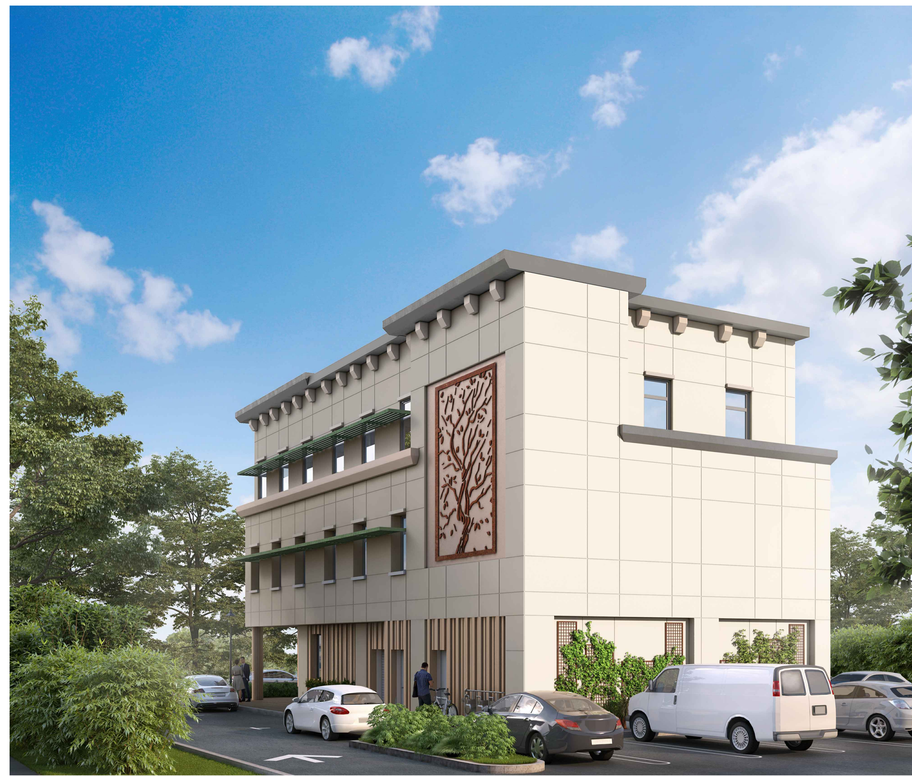
VIEW FROM HOPE STREET PARKING LOT 6
