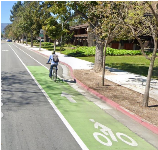
Figure 4: Class II Bike Lane (conventional bike lane left; buffered bike lane right).
