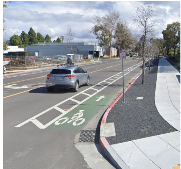
Figure 4: Class II Bike Lane (conventional bike lane left; buffered bike lane right).
