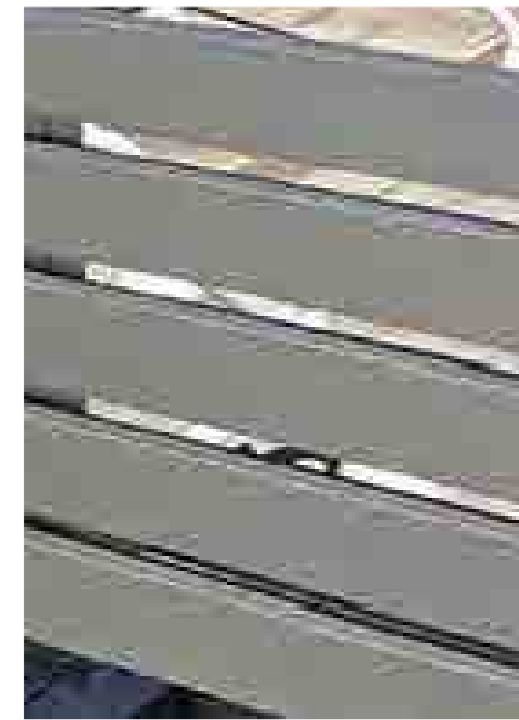
(MS) LOUVERED METAL ROOF SCREEN, CASCADE ROOFTOP SCREENS, COLOR: SLATE GRAY
