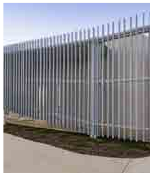
(MF) ALUMINUM METAL FINES @ PARKING GARAGE
