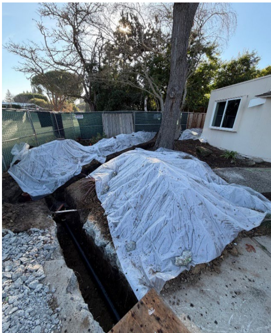
Photo #5 Trench for sewer line
