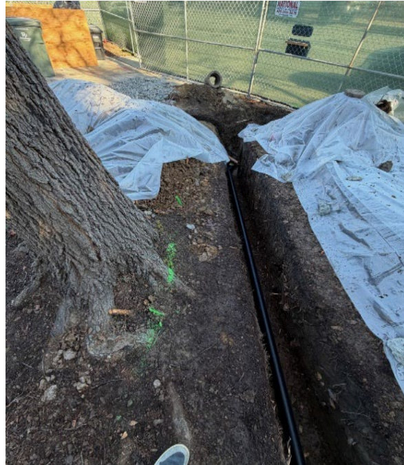
Photo #6 – 2-foot distance from trench to tree
