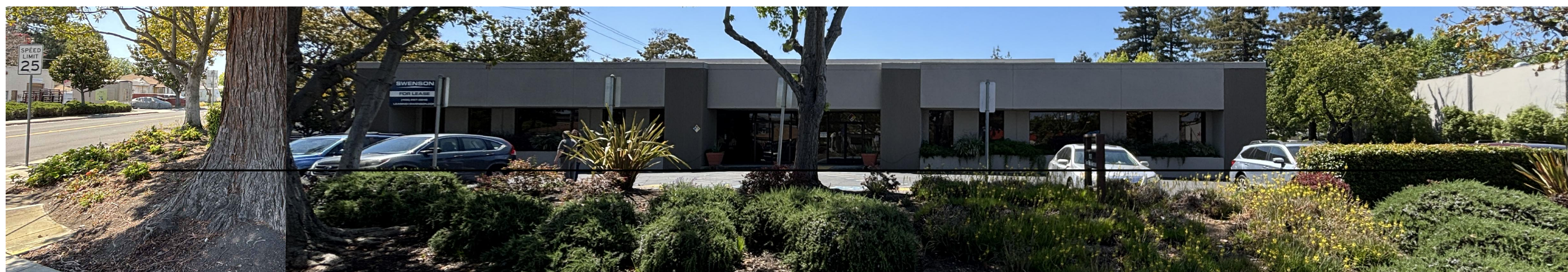
North Elevation photos
