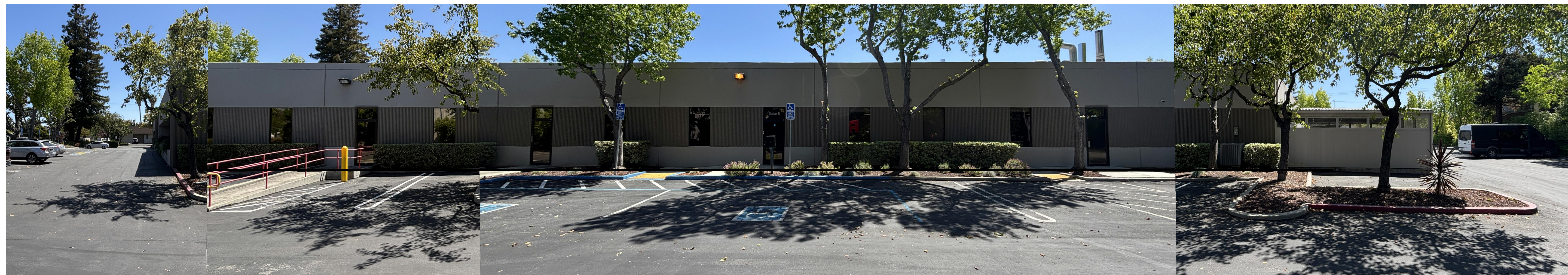
West Elevation photos
