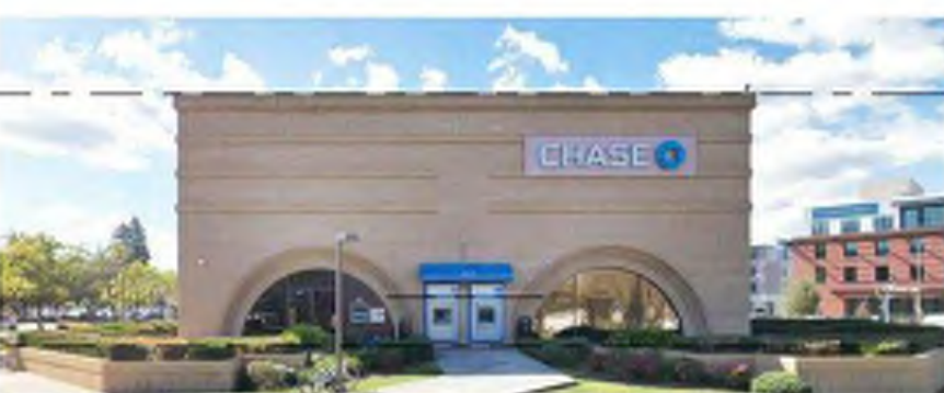
EXISTING CHASE BANK (REMOVED) - ATM SIDE
