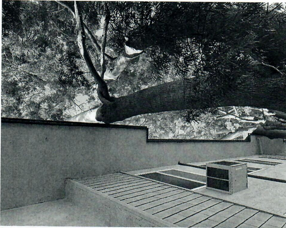
Picture 13: Top of existing tree No. 2 in contact with roof framing system
