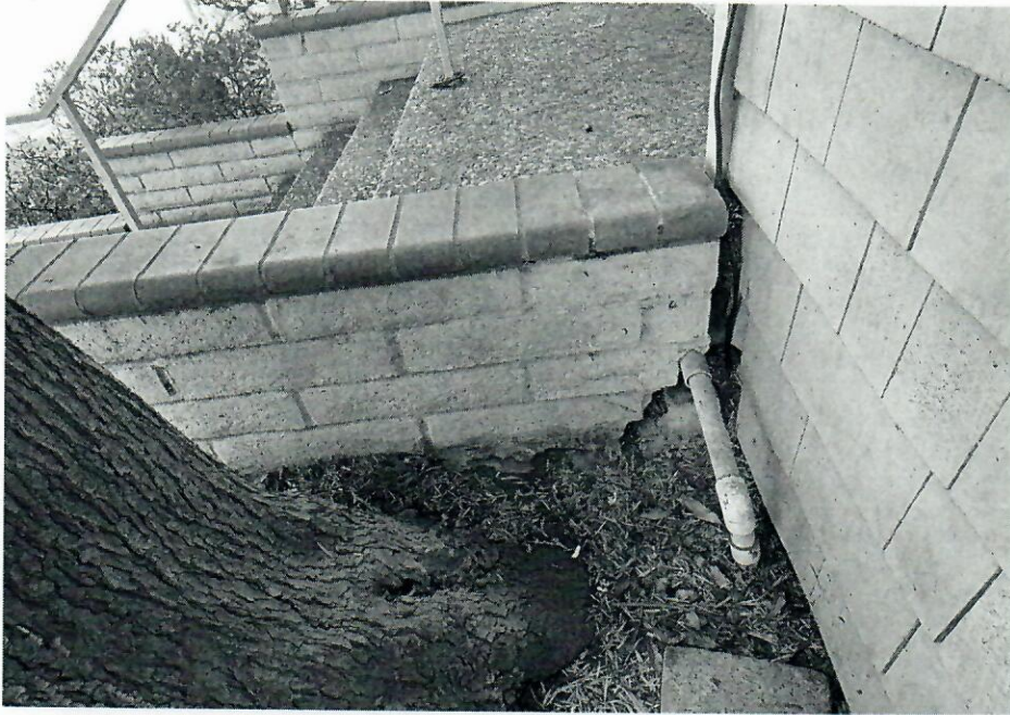
Picture 11: Location of short step wall separation from building
