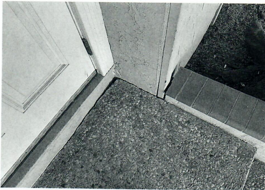
Picture 10: Location of landing tilt at corner
