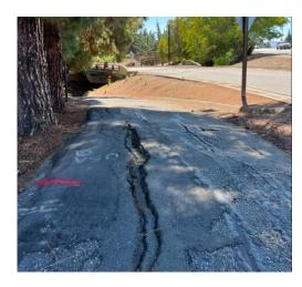
Figure 1: Existing Poor Asphalt
