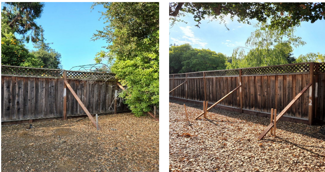
Figure 2: Existing Fence Condition
